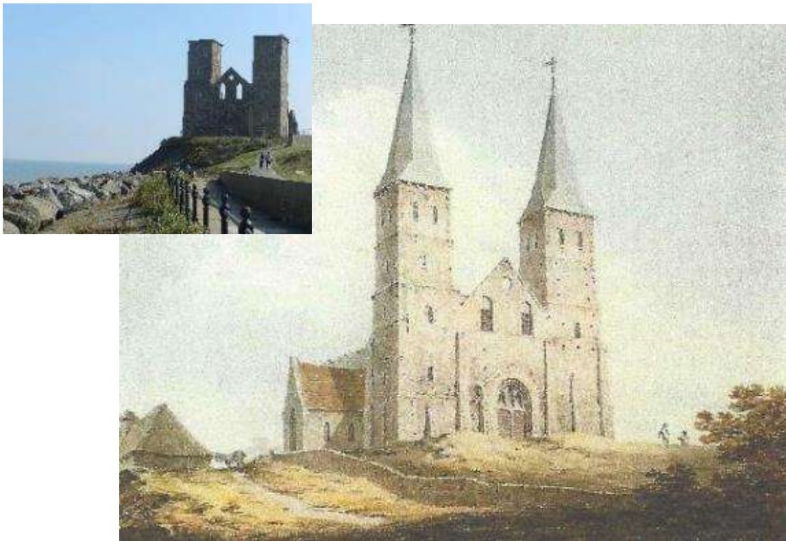
Figure 3B40. 'The Reculver', commonly called 'The Two Sisters' by James Malton, 1798. Malton's watercolour drawing shows a building existing between the seaward side of the church and the cliff edge. Image: Courtesy Bonham's. Private collection.
