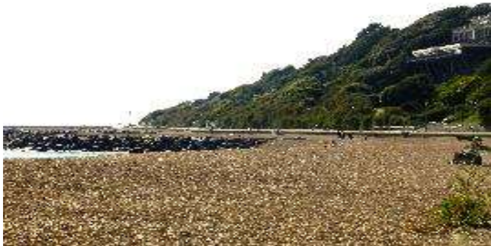
Figure 3B153. The present day view, shows the coastal slope, which has faced some instability problems and the upgraded coastal defences including rock groyne.
