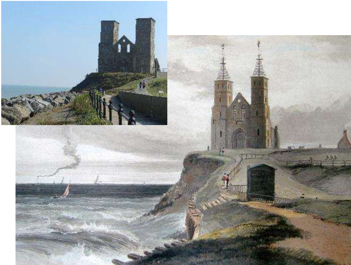
Figure 3B7. Reculver Church', North Kent coast by William Daniell, RA engraved in 1824. Some rudimentary coastal defences can be seen, which were helping to preserve this important landmark for navigation. A substantial rock revetment now protects the site.
