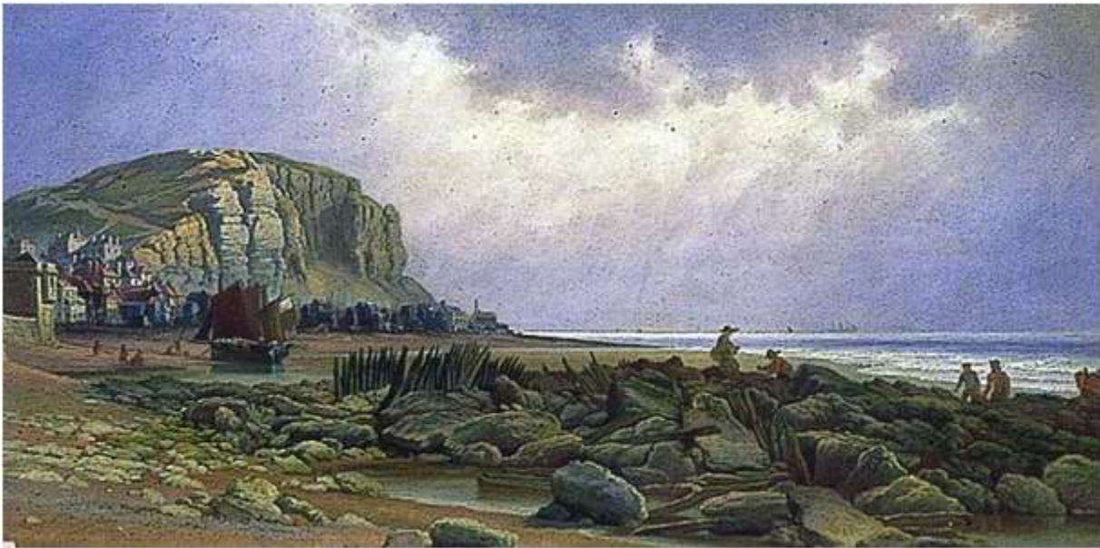
Figure 3C10. 'Remains of the Elizabethan Harbour at Hastings' by Charles A. Graves, 1901. This view shows the timber relics of the harbour. Beyond is the fishing village and behind it the jointing and mechanisms of failure of the rugged sandstone cliffs are particularly well painted, Image courtesy Hastings Museum and Art Gallery
