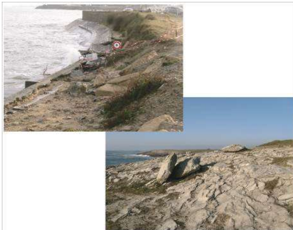
Figure 3K21. Natural threats on the Quiberon coasts, (top): damages on the Penthièvre dyke after a storm, (bottom): damaged Neolithic site of Kerné (cl. Le Pessec 2011).
