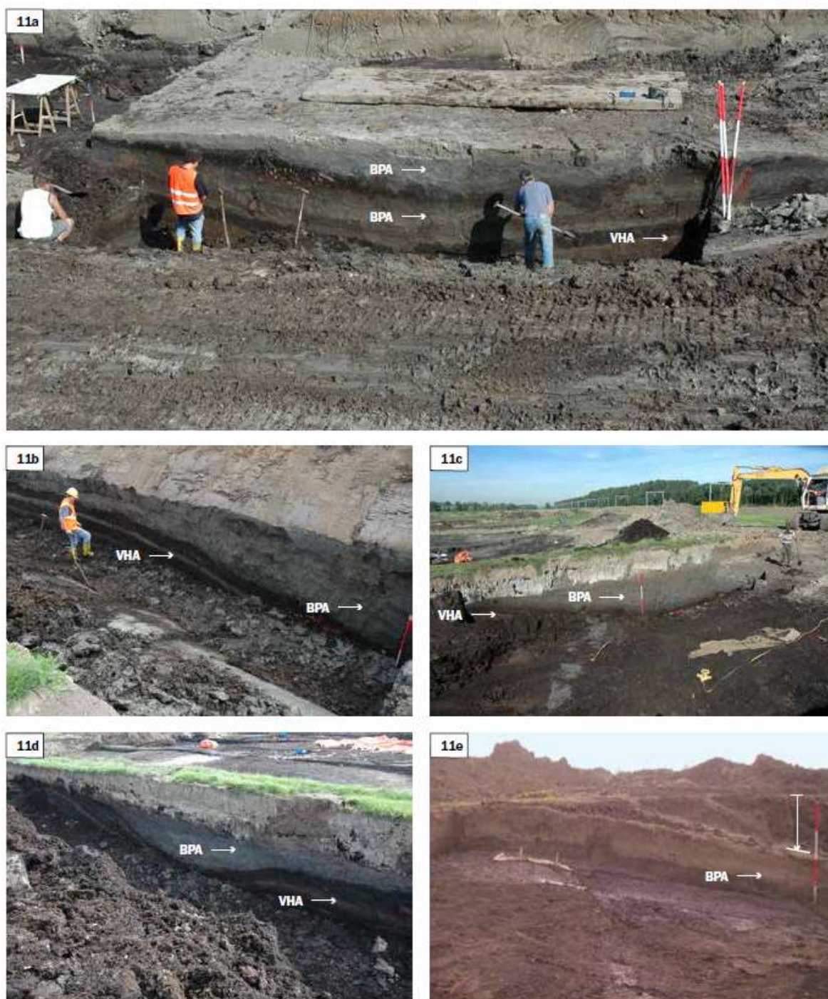
Figure 3N28: Picture of differential subsidence of the BPA clay layer caused by autocompaction of the peat which was induced by gravitational forces during the clay deposition of the BPA layer. Figure 3N28a. Loading structure of the BPA clay. The Medieval peat (Hv-1), only found below the loading structure, is not affected by oxidation because the peat layer was come down below the groundwater level, in find location area Vz02 in sector West. Figure 3N28b. Loading structure of the BPA clay on top of the Hv-3 peat layer. The BPA clays are the lateral deposits of a creek, in find location area Vz07 in sector East; Figure 3N28c. Loading structure of the BPA clay on top of the Hv-3 peat layer. The BPA clays are the lateral deposits of a creek, in find location area Vz09 in sector East. Figure 3N28d. Depression caused by loading of the BPA clay in the Hv-3 peat layer, in find location area Vz09 in sector East. Figure 3N28e. Subrecent loading of the BPA layer in the Hv-3 peat layer, after the removal of the central ground depot of the excavation in 2005, the maximum subsidence of the surface level was more than 1,5 m, in find location area Vz01 in sector West.
