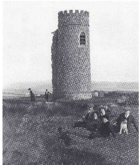
Figure 4.23. (above right): A photograph of the tower even closer to the cliff edge. If the height of the structure is known an assessment can be made from paintings and photographs of the distance to the cliff edge (photograph courtesy of N. Storey).
