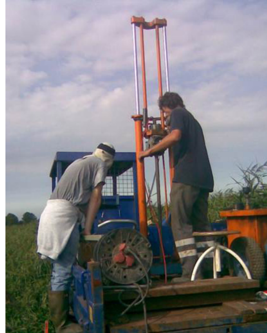
Cone penetration testing in the Scheldt polders (Image courtesy of T. Missiaen, Ghent University).
