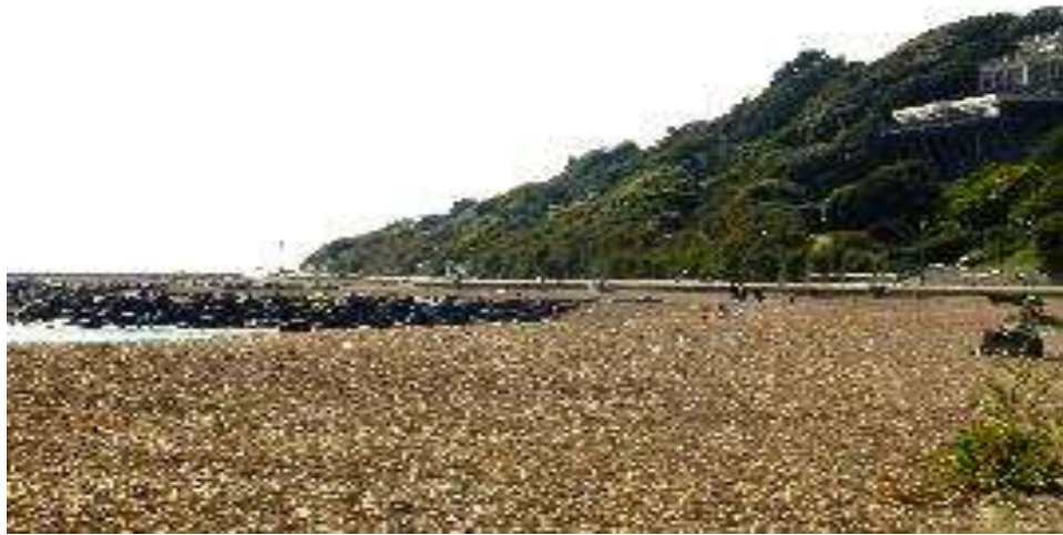
Figure 3B153. The present day view, shows the coastal slope, which has faced some instability problems and the upgraded coastal defences including rock groynes.
