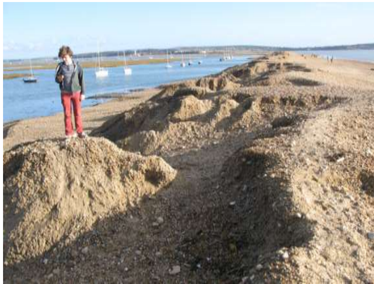
Figure 3D.2: Damage caused by the storms in January 2014
