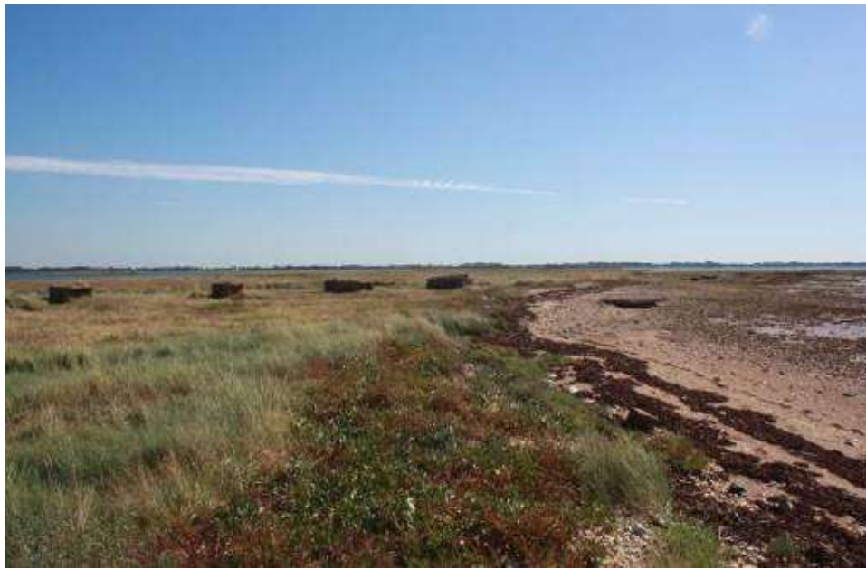
Figure 3D.58: WWII decoy structures on Baker's Island. Structure on the beach are now being eroded.
