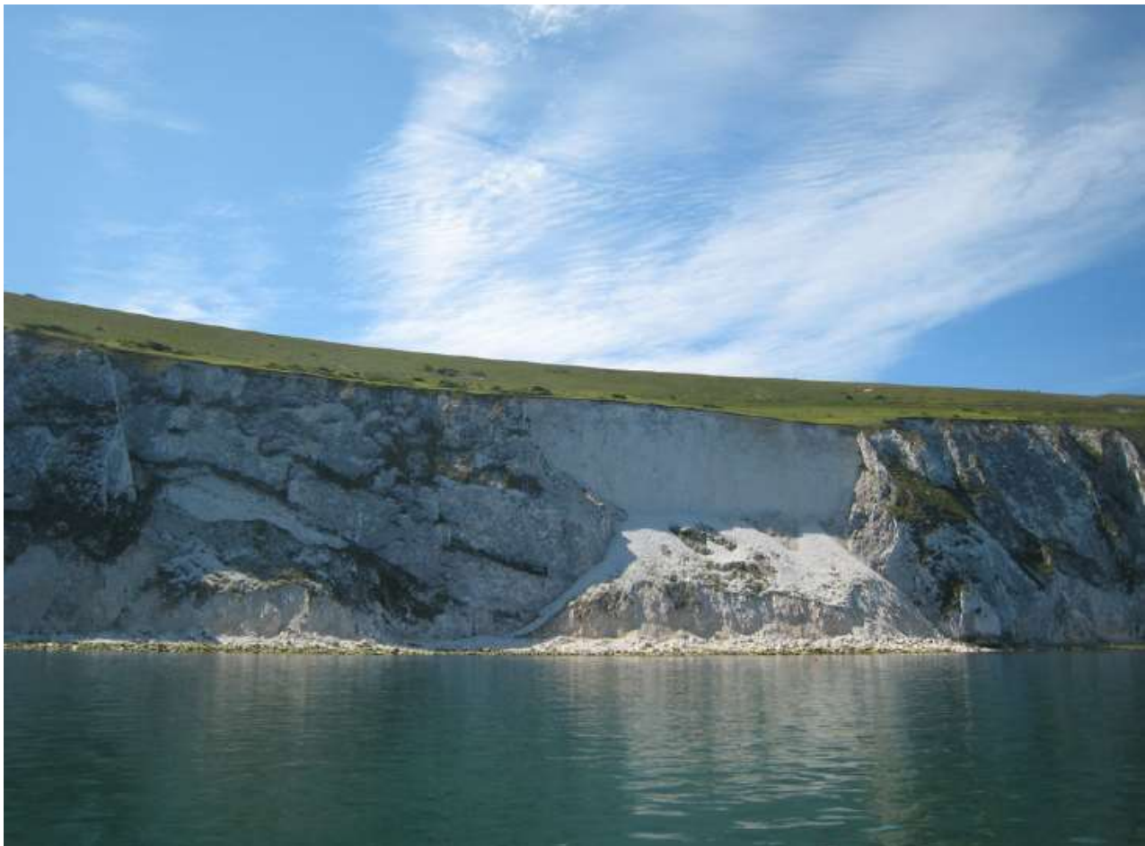
Figure 3D.49: High chalk cliffs characterise the shoreline along the southern side of Alum Bay and are subject to on-going erosion resulting in significant landslips (Photo: Ine Demerre)
