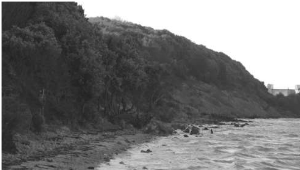
Figure 3D.11: Active erosion and rotational sliding forming a cliff along the north edge of Victoria Country Park.
