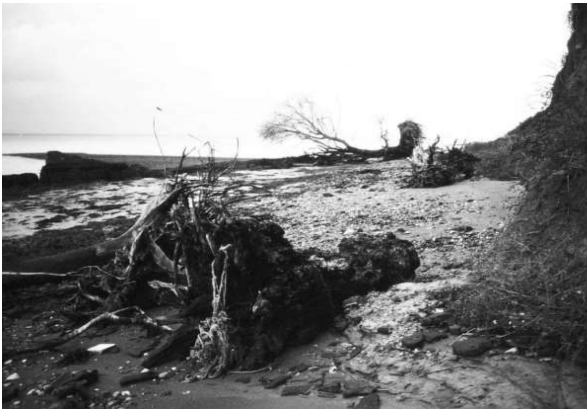
Figure 3D.12: Fallen trees below Bouldnor Hill resulting from cliff erosion
