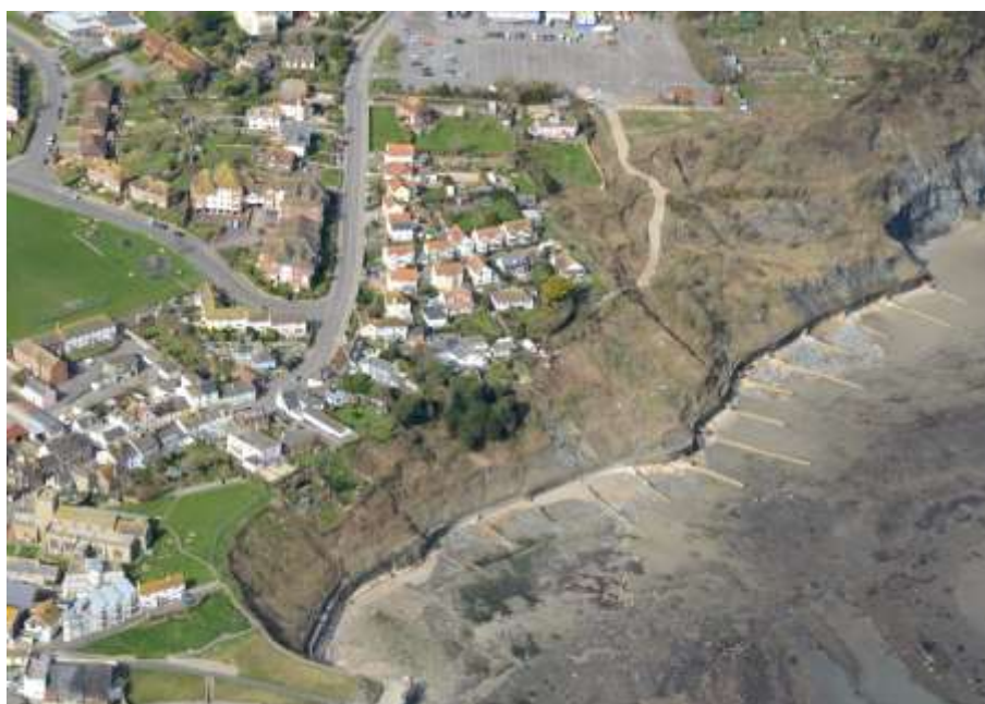
Figure 3E3: East Cliff at Lyme Regis. Coast and cliff protection and drainage works are currently in progress in order to reduce risks for cliff top properties and assets. Photograph courtesy Halcrow CH2M HILL.
